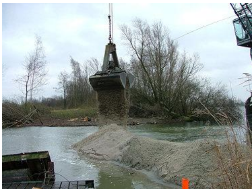
Figure 2: Construction of dams at “Het Groene Eiland”
